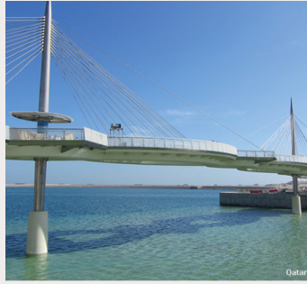
Pasarelas de Lusail. Victor Gómez. Pedestrian bridges in Lusail.
